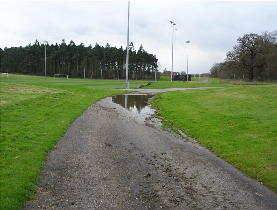
Photograph 12: Road drainage swale
