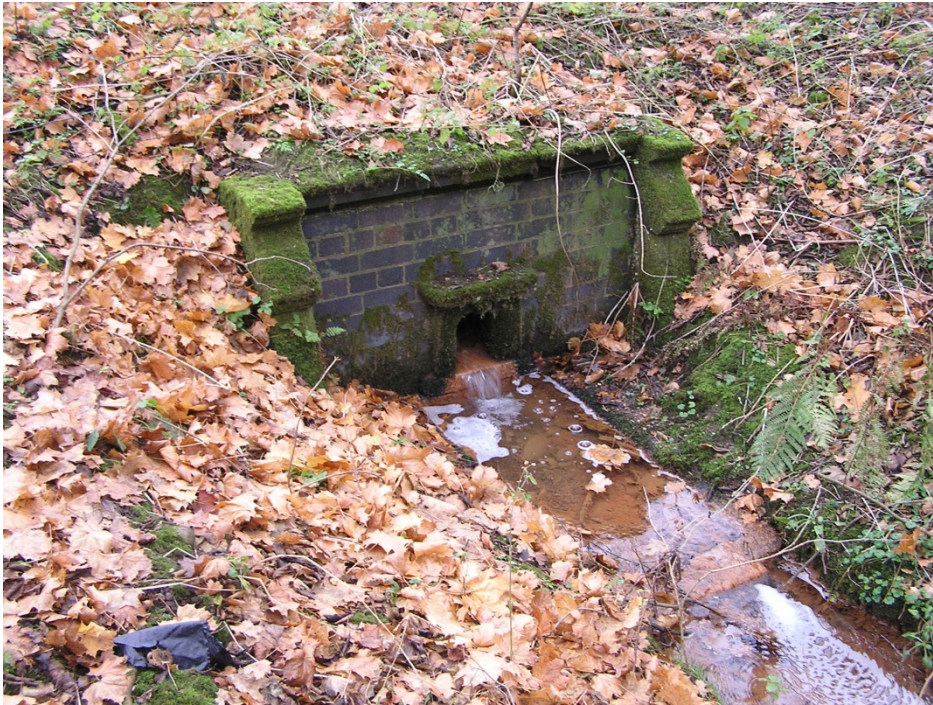
Photograph 13: Land drainage outfall to Lin Brook
