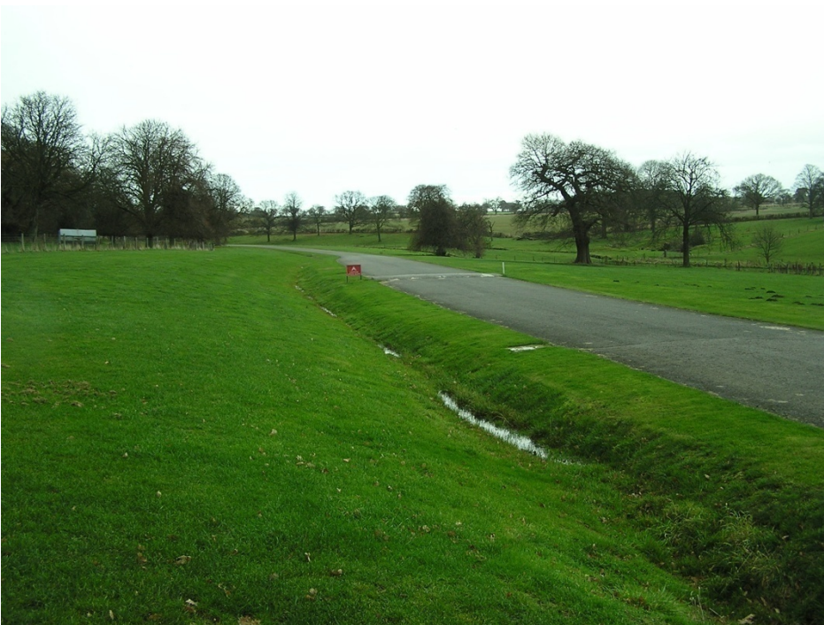
Photograph 12: Road drainage swale
